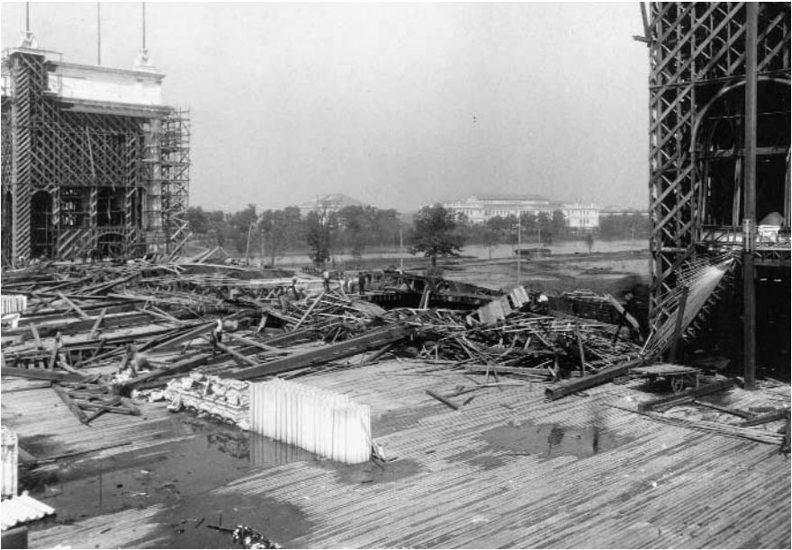
Manufactures and Liberal Arts Building, after the storm of June 13, 1892.
